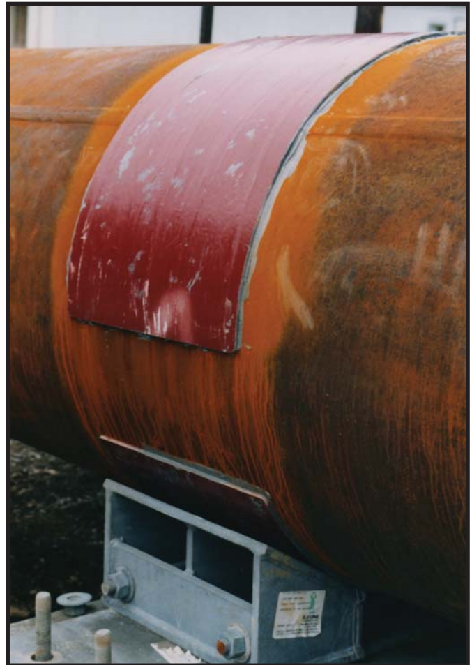
TYPE #120 Spacer & Type #180 Saddle Prior To Painting and Installation Of Hold Down Strap
