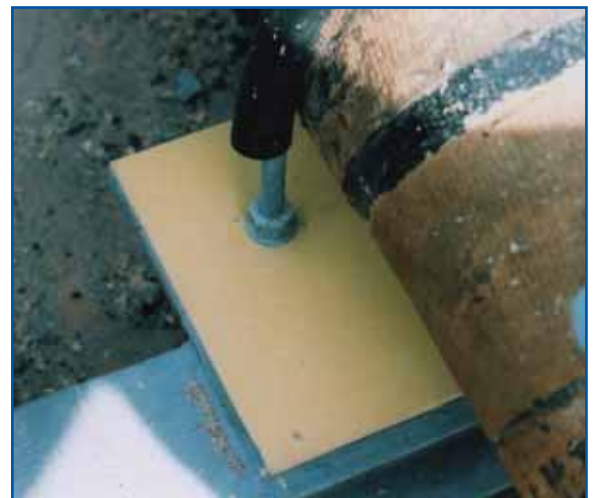
1/4” FRP FLATTIE being used to prevent contact between gas main and bridge support.
