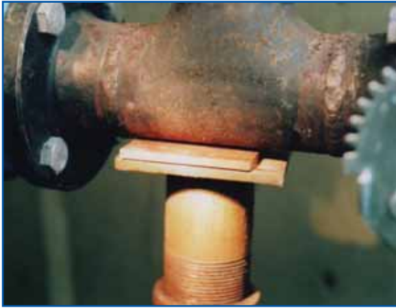
Isolate valves from supports.
